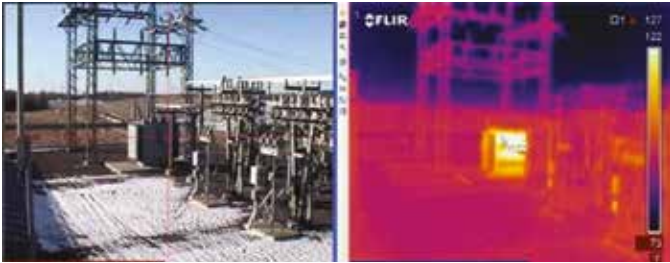
Digital photo and thermal image of a substation showing a transformer with excessive temperature.
