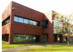
FLIR Systems, Portland
